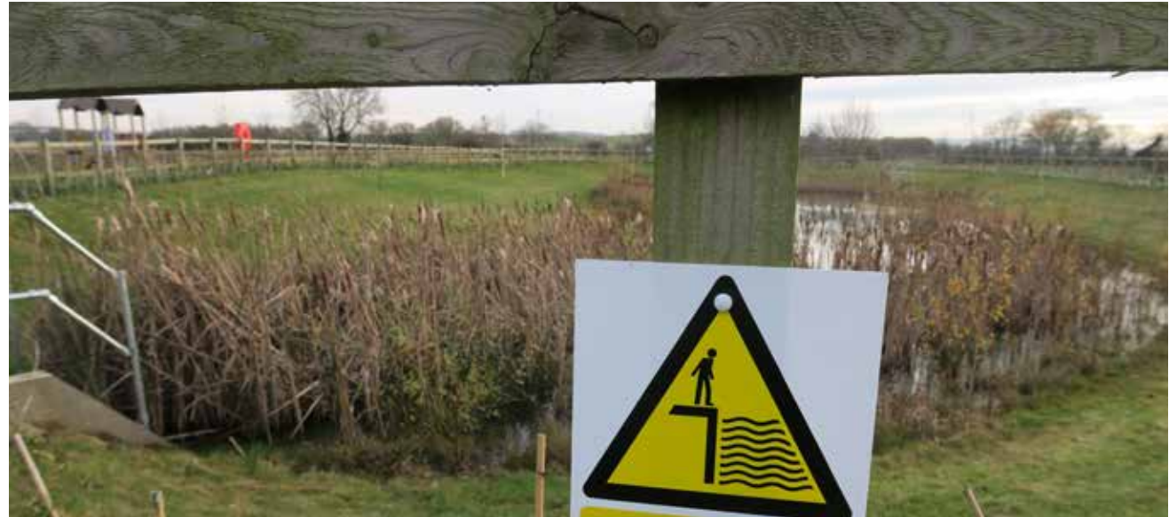
Figure 80: Attenuation ponds and detention basins must be integrated into the green space strategy and designed with safe public access in mind so that they do not necessitate fencing. Designs similar to the facility in this picture must be avoided because they are dangerous and have unattractive fencing.
