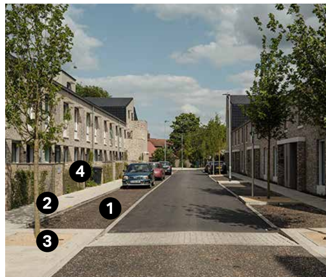
Figure 68: A good practice example - on -street inset parking, Goldsmith Street, Norwich.
