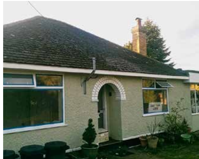
Figure 32: The majority of houses in the area are detached, but bungalows can also be found along the road, Fisher Row.
