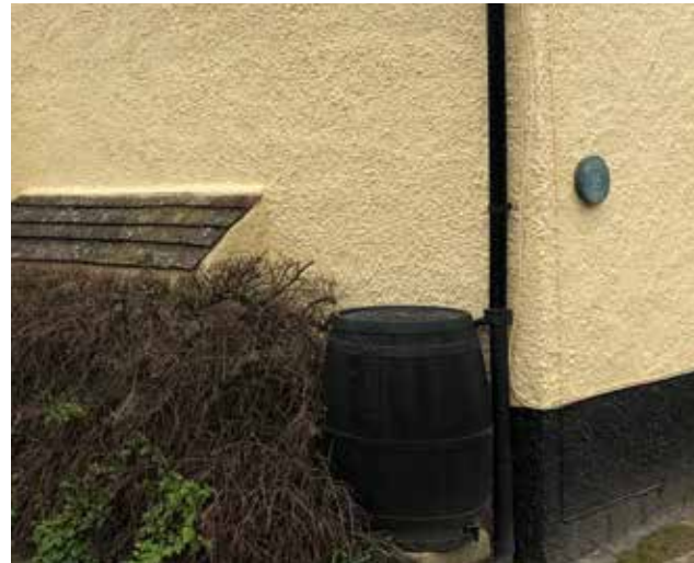
Figure 85: Examples of water butts used for rainwater harvesting in Reach, Cambridgeshire.
