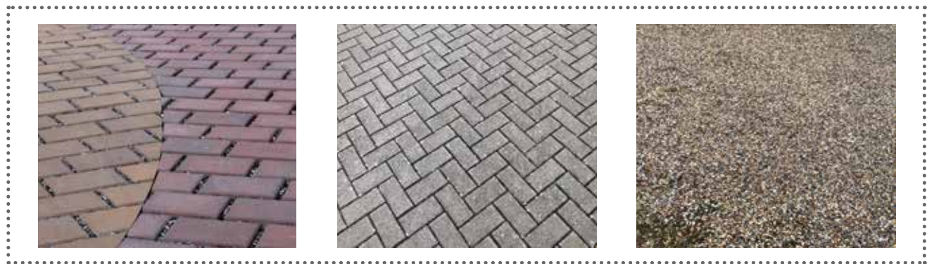
Figure 91: Examples of permeable paving treatments: unbound clay pavers (left), precast concrete setts (centre), and gravel (right).
